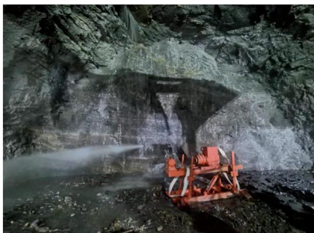
Fig. 2. Water inrush situation of the tunnel face.
