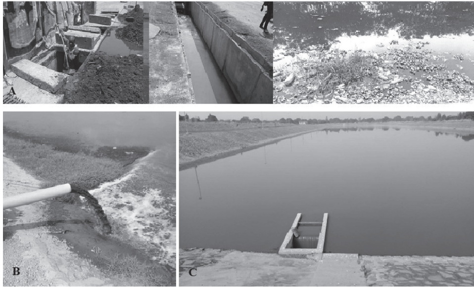
Fig. 4. Wastewater collection systems and treatment in Burkina Faso. A. canalization of wastewater, B. wastewater influent, C. wastewater effluent.
